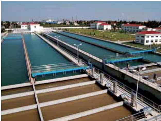
Jiangsu Changshu Water Plant
