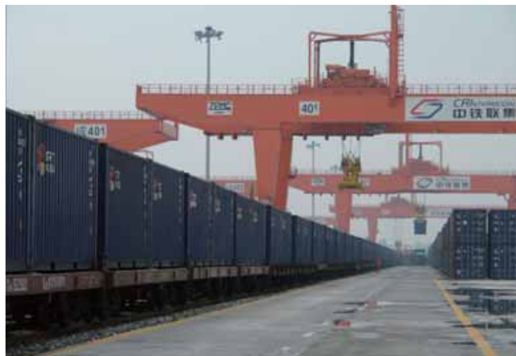
Chengdu Rail Containers Terminal
